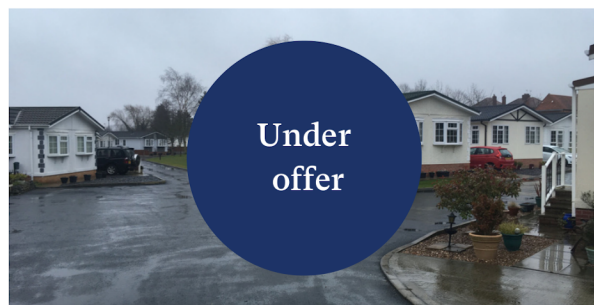
Residential mobile home park, Nottinghamshire (Ref:YRK1922)
